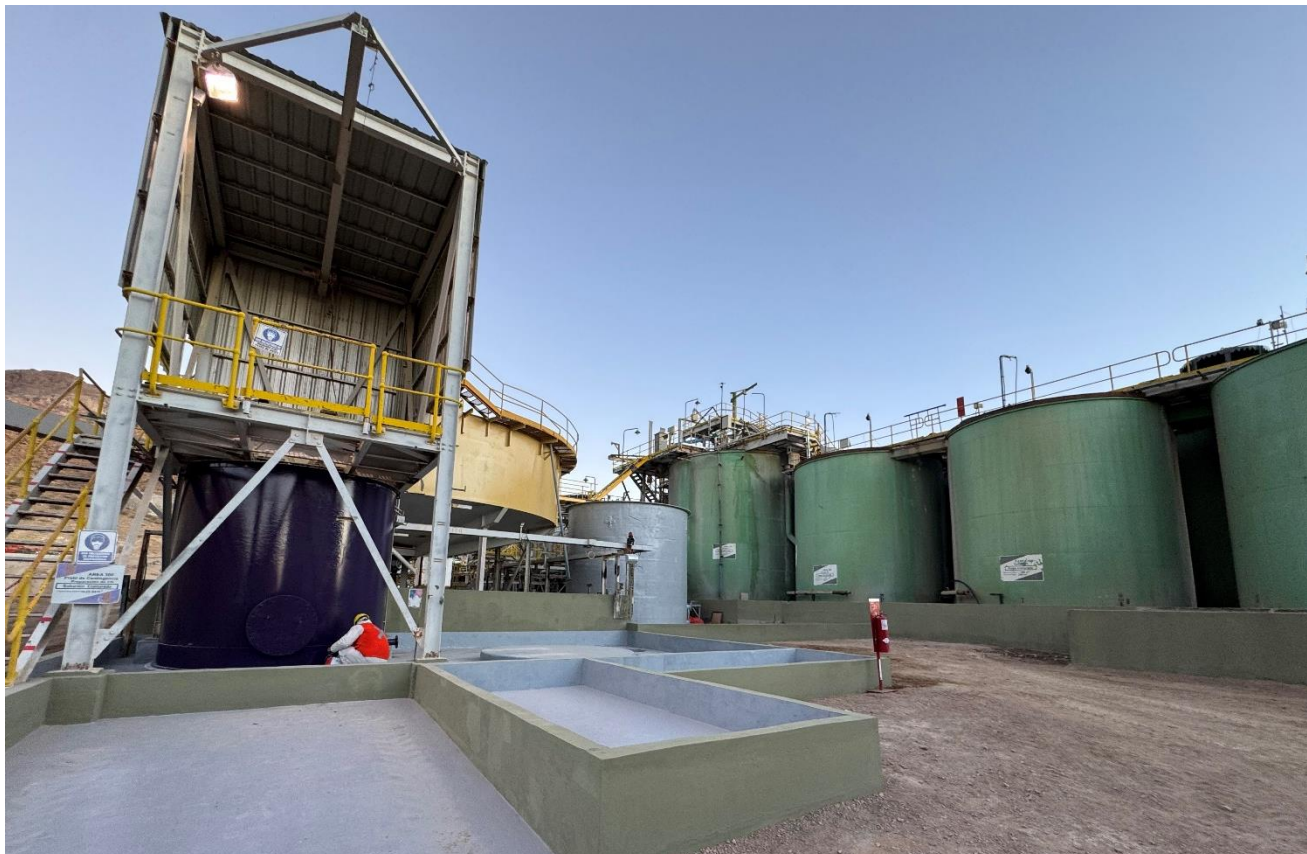
Figure 3: Leaching Tanks (Area 300)
