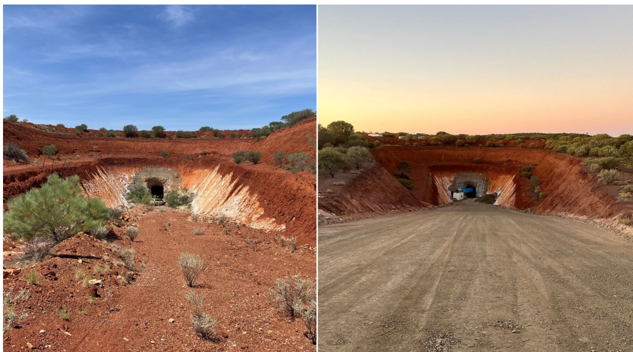
Figure 8: Refurbishment of K2 boxcut and portal
