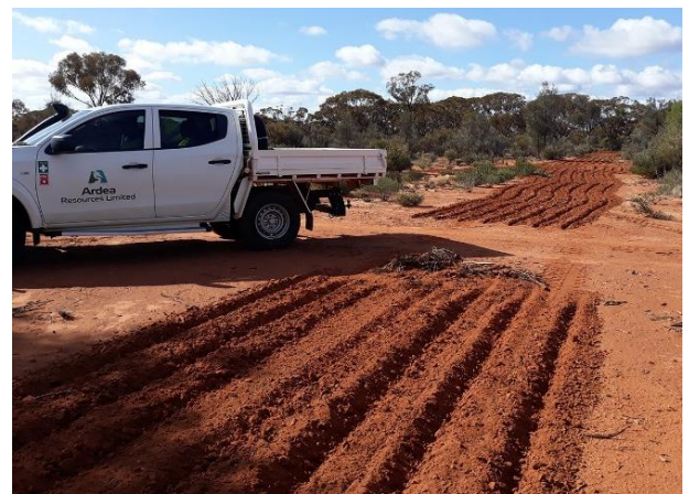
Figure 9: - left: Planned Goongarrie Hub in-pit tails disposal and rehabilitation strategy. Above- Showing scarification of disturbed areas, during rehabilitation of Goongarrie South drill sites.
