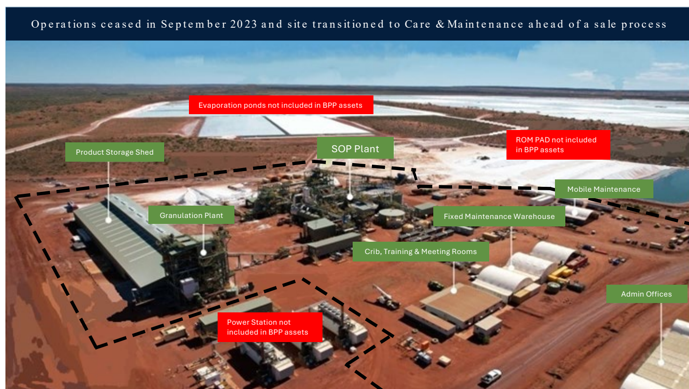
Figure 1 – Photograph of the Beyondie Potash Project in 2023 when in operation by Kalium. The Transaction comprises a fully constructed processing plant, site offices and maintenance infrastructure. Specific plant components include, KTMS crushing circuit, Kainite conversion circuit, column flotation circuit, liquor cooling heat exchangers, evaporative cooling circuit, product separation centrifuges, SOP recovery and granulation units, RO water plant and a bulk storage shed.
