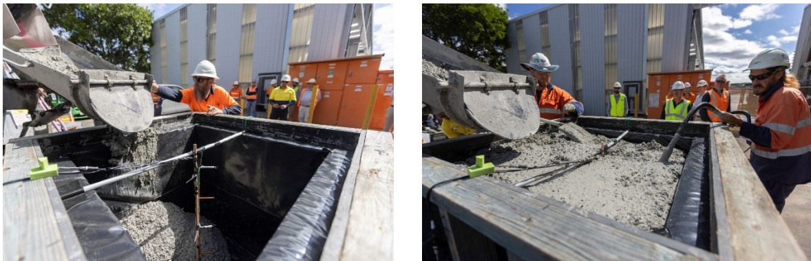
Figure 2: Concrete hotbox demonstration pour and temperature monitoring
