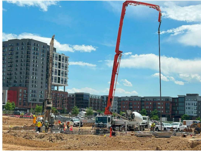
Figure 8. Pouring concrete for caissons
