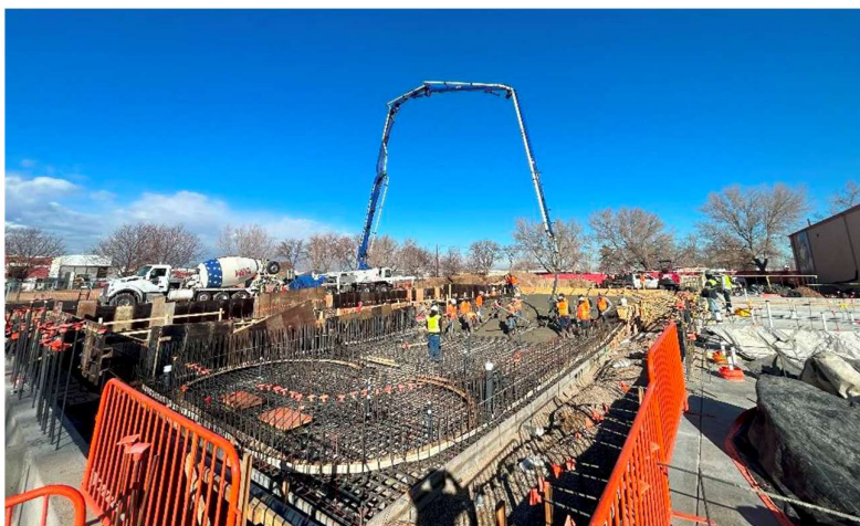
Figure 10. Pouring Concrete - Swansea Recreation Centre Swimming Pool
