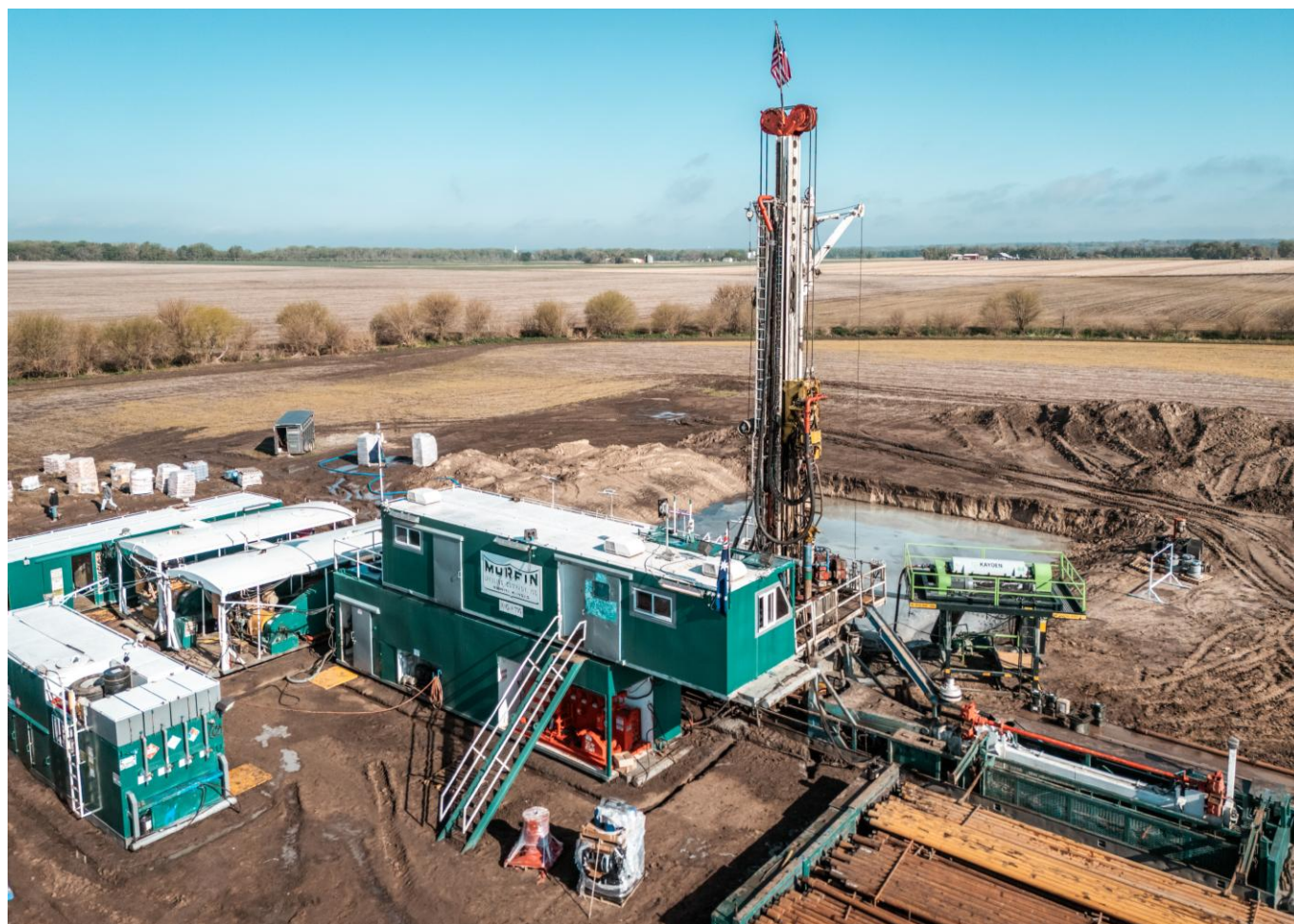
Figure 2. Murfin 116 rig drilling at Sue Duroche 3 well site, Kansas, USA.
