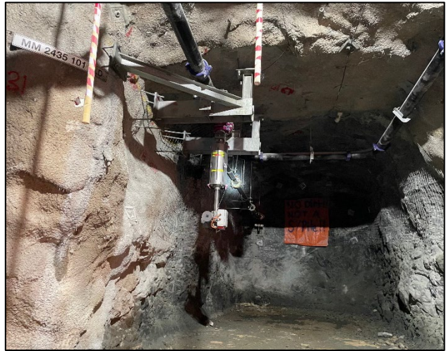
Figure 5: Underground Paste reticulation
