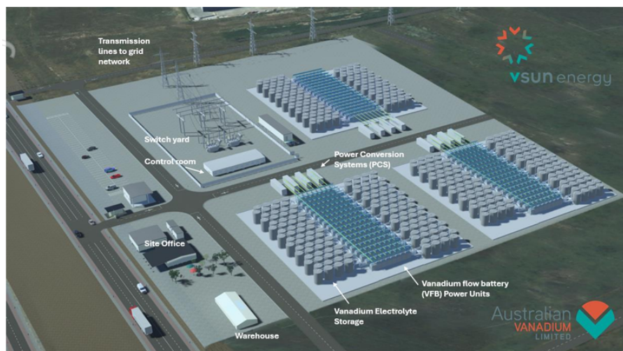
Figure 4 – Project Lumina: a turnkey VFB BESS architecture tailored for Australian build-own-operate delivery
