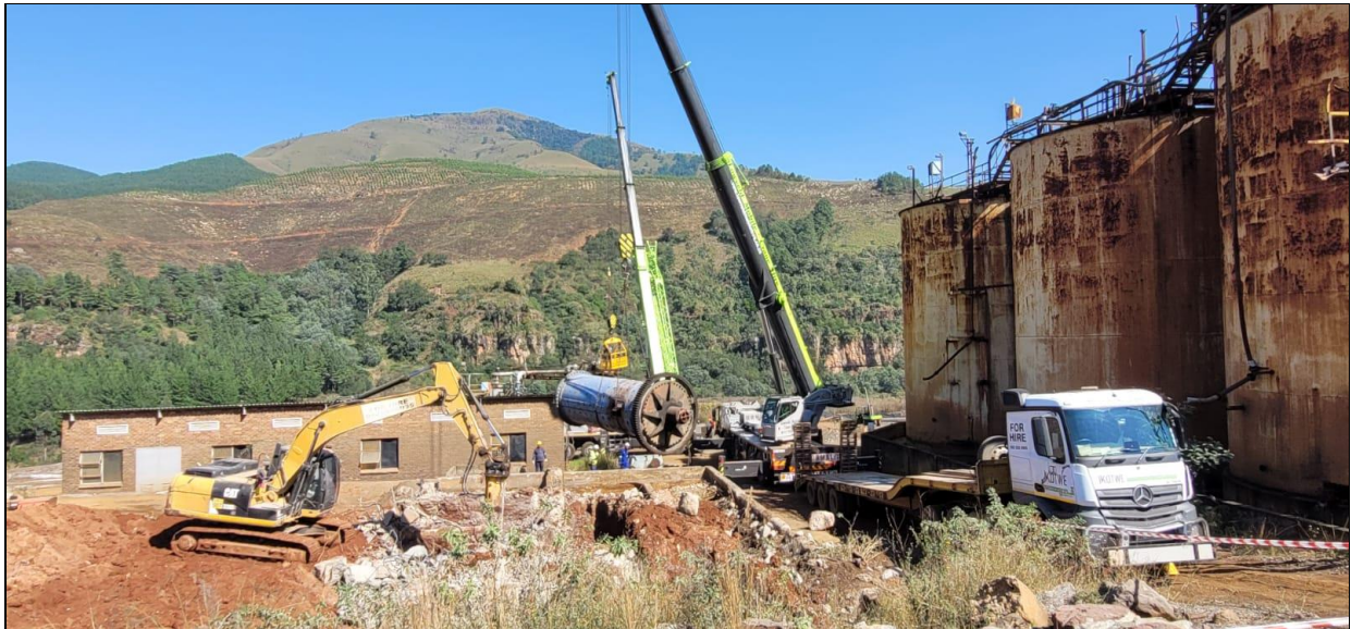
Figure 5: Breaking of old mill civis and loading of ball mill
