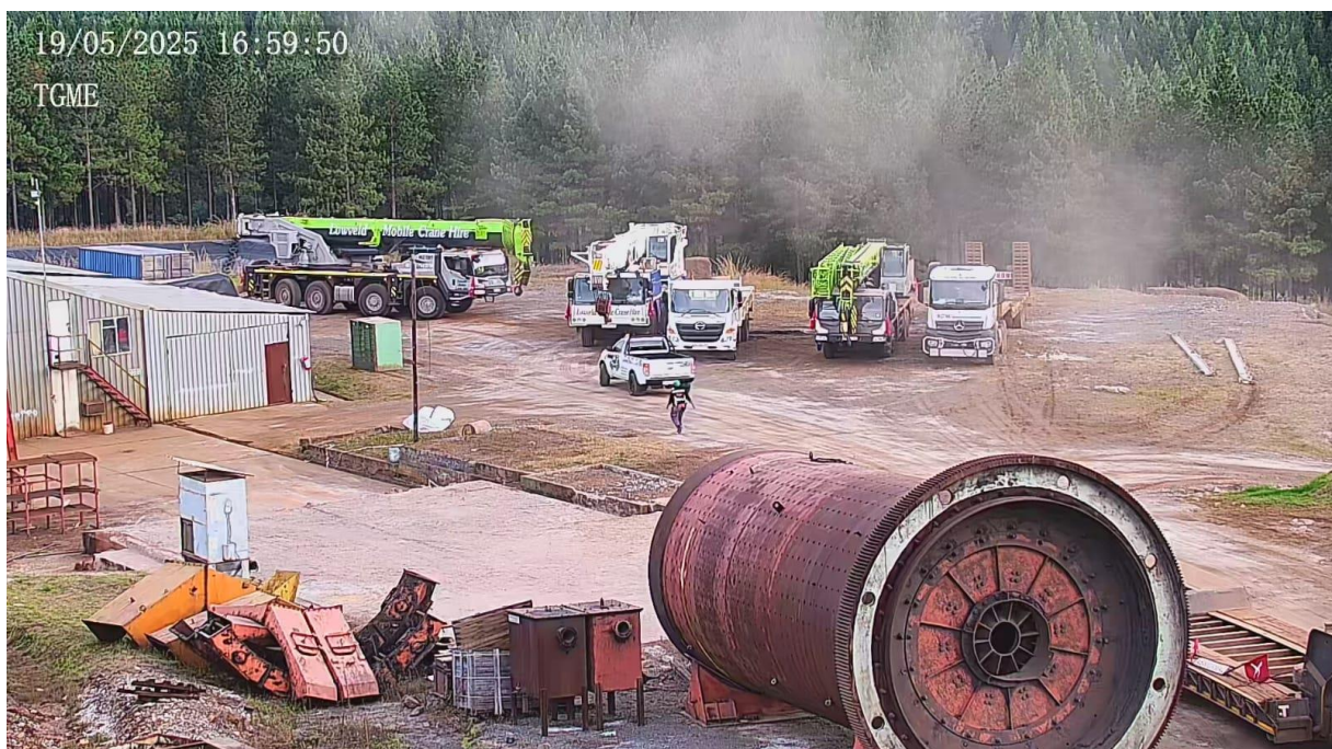
Figure 2: Mobile Cranes and Flatbed Trucks assisting in deconstructing the old plant.
