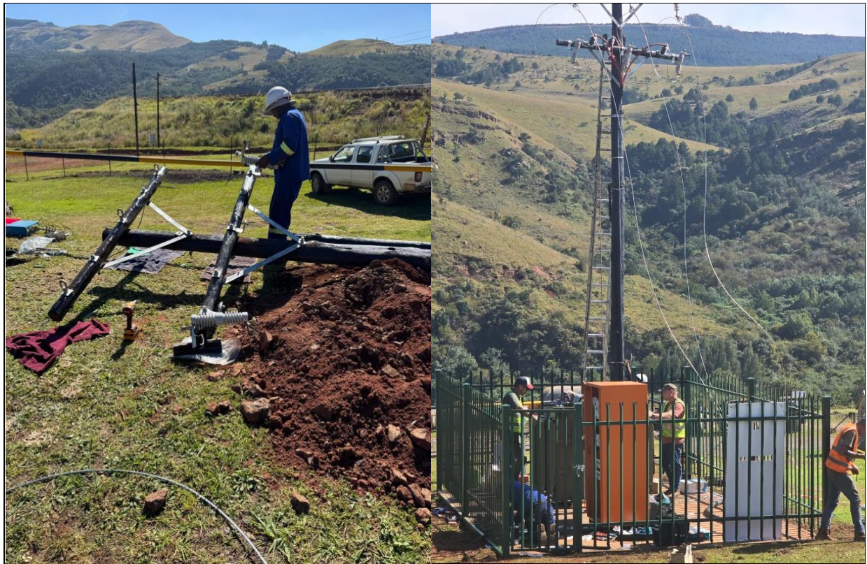
Figure 4: Installation of temporary electrical plant supply
