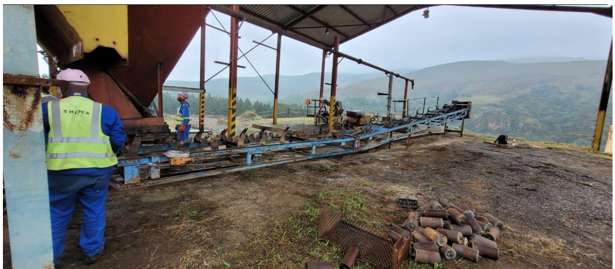
Figure 11: Removal of old conveyor belt structure
