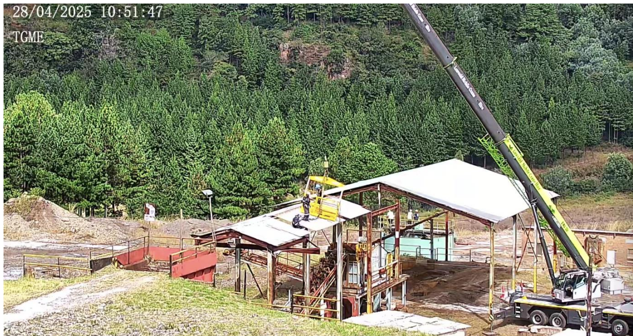
Figure 9: Removal of old mill sections
