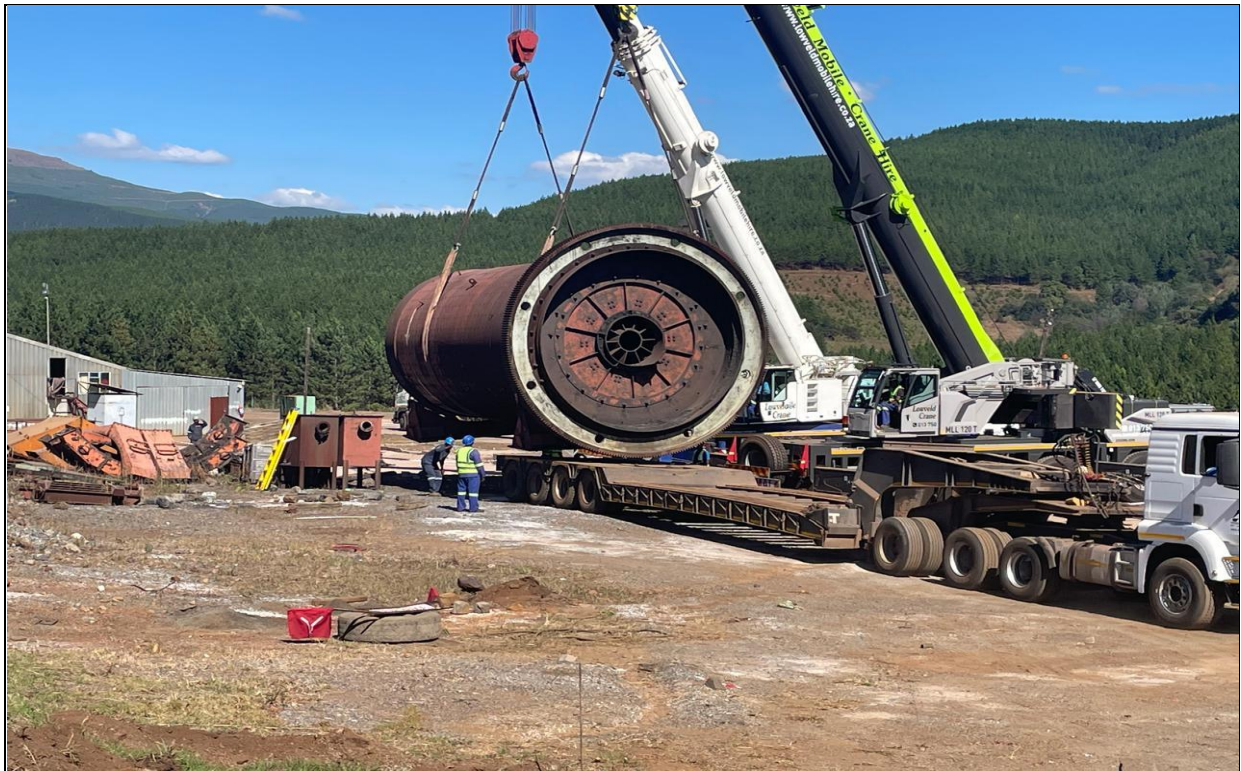
Figure 6: Lifting and loading of the big ball mill for transport to the laydown area
