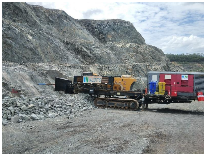
Depressurisation hole drilling
