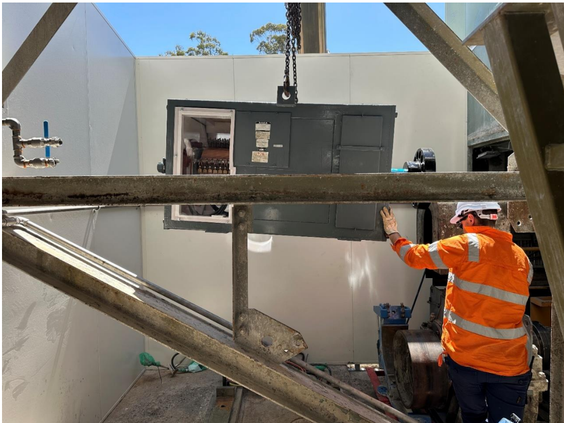
Figure 7 – DC mill motor installation
