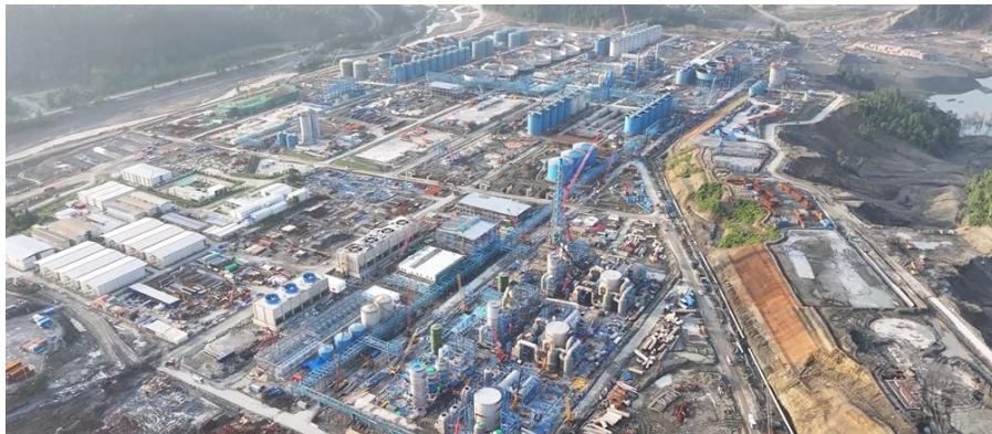
HPAL smelter with integrated sulphuric acid and power plants shown in the foreground
