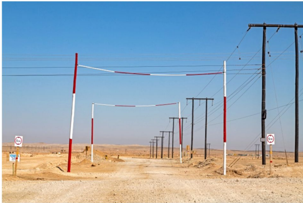
Figure 4: Power grids on site now live with safety precautions to prevent vehicles crossing under installed lines
