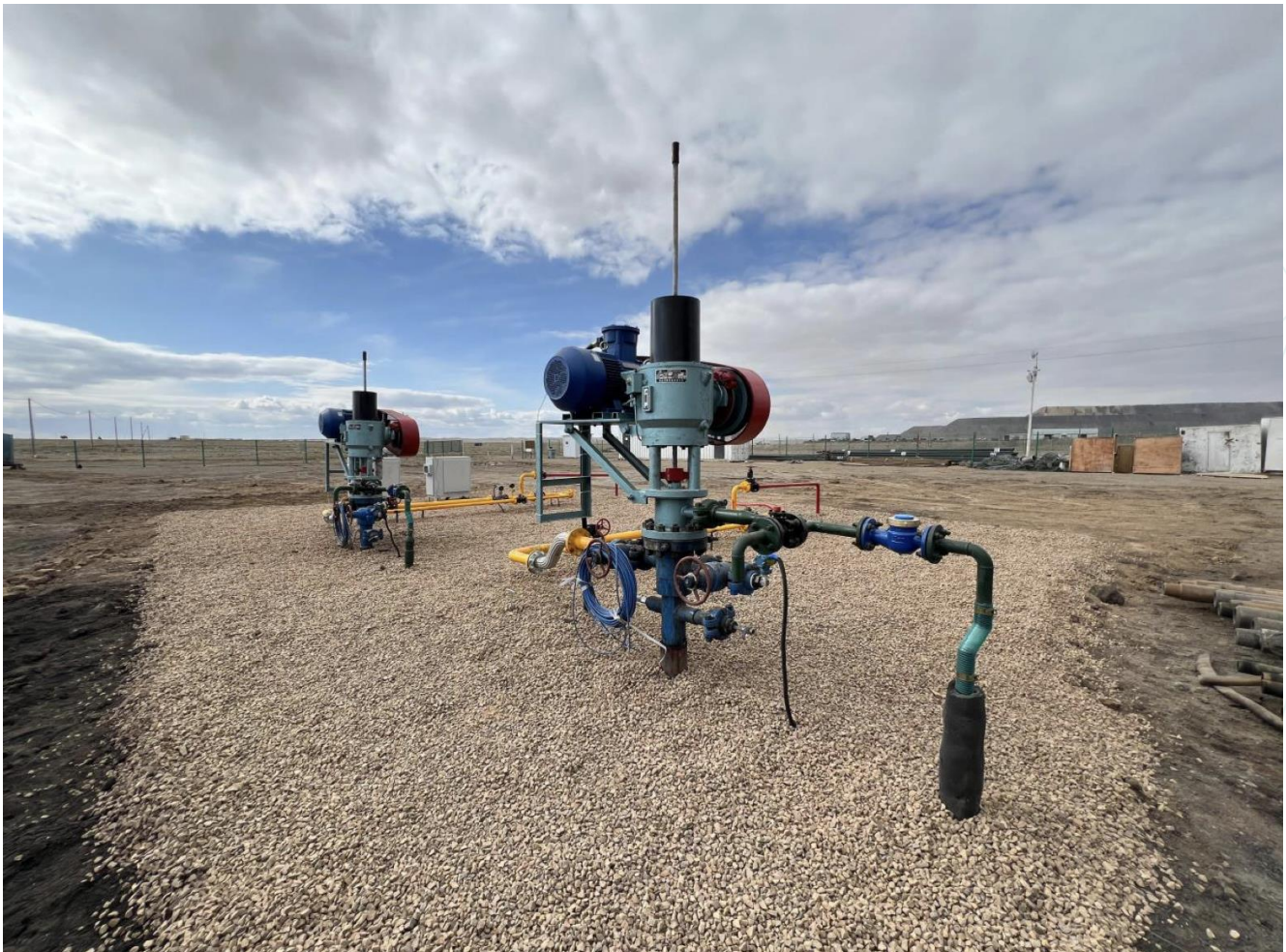
Figure 3: Completed CBM Gas Production Wells at the Red Lake field
