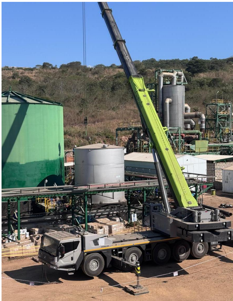
Figure 6: Placement of new acid dilution tank
