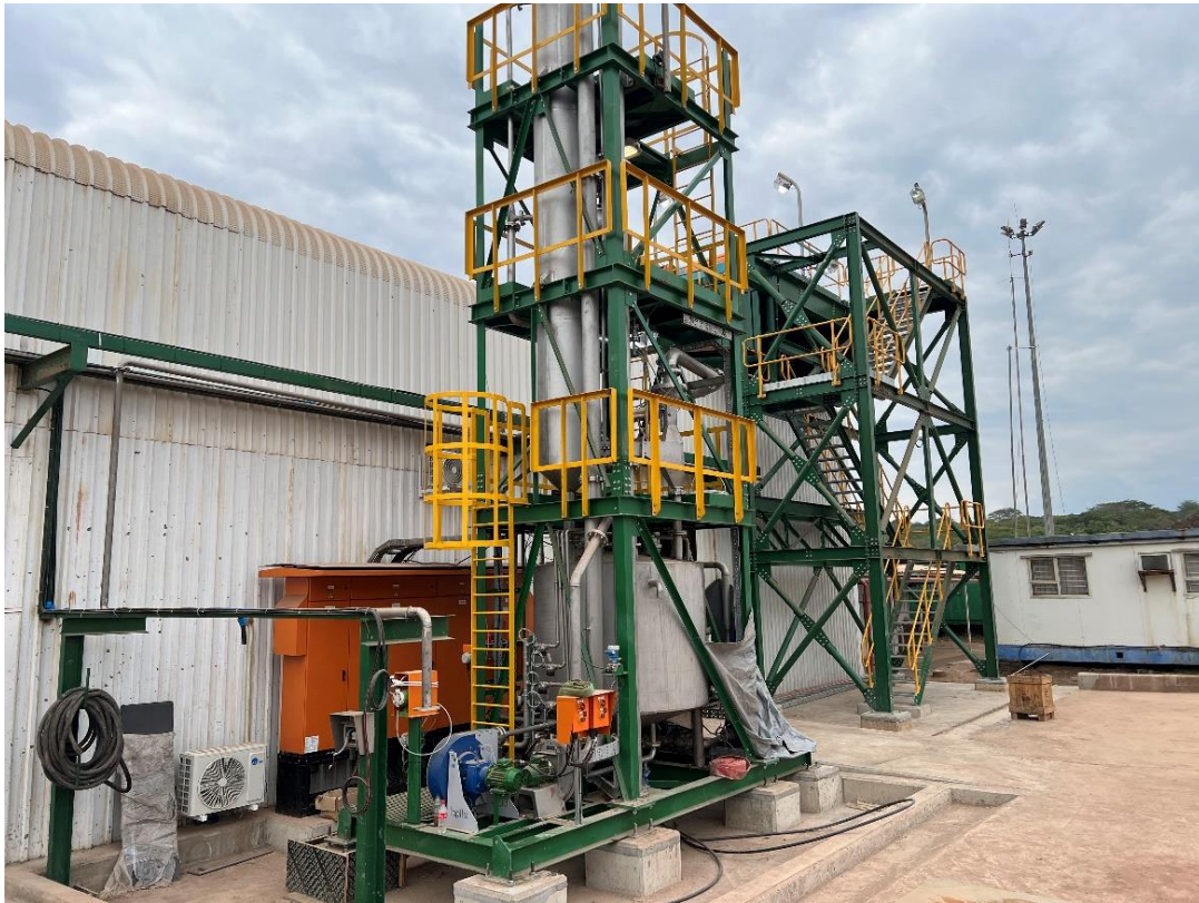
Figure 7: New off-gas scrubber installed outside the drying and packaging building
