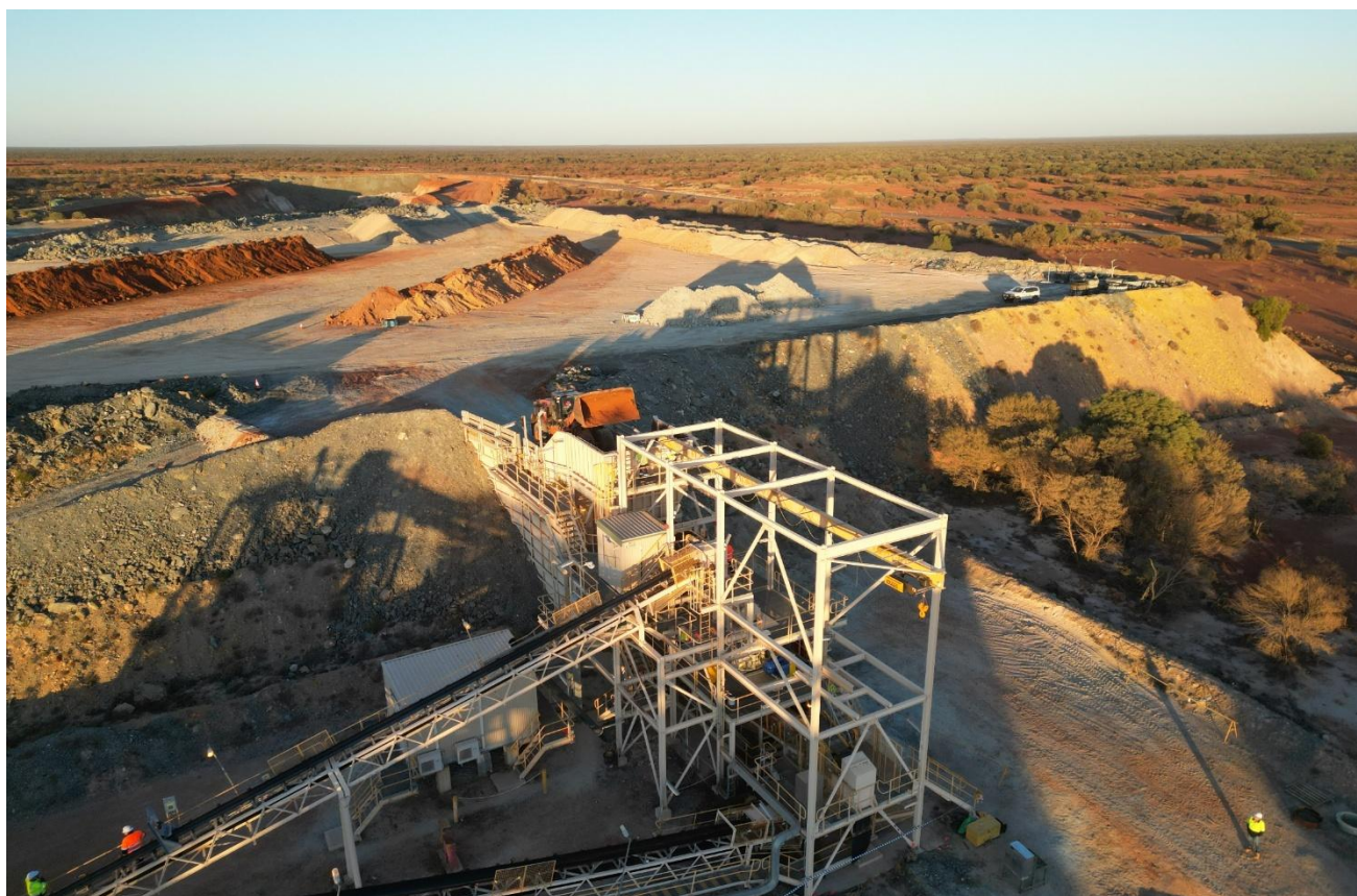
Figure 2: First ore being fed into the crusher, 11 June 2025.
