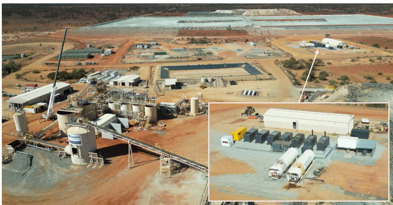
Figure 3: Power station upgrade completed.
